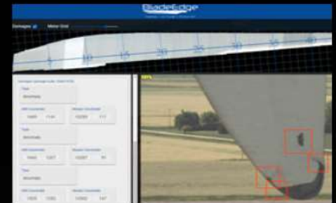
WIND TURBINE INSPECTION
